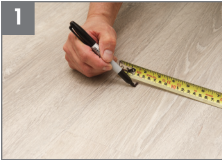
1 Measure 1-1/2" inside the perimeter of the damaged plank, and mark.
