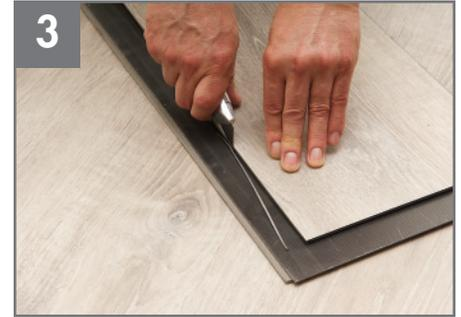
Remove the long, tongue edge of the replacement plank.
