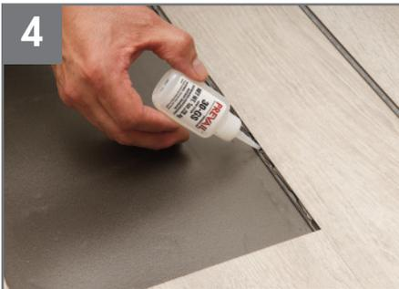
Apply a scant bead of Prevail™ 30-GS to the exposed groove sides of the flooring surrounding the repair.
