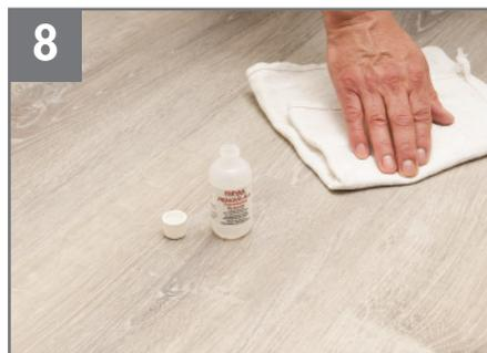
Remove excess adhesive immediately using a small amount of Prevail™ Remove-All applied with a clean, white lint-free cloth. Never pour directly onto the floor.
