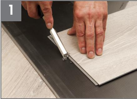
Remove the lock on the long and short sides of the replacement plank.
