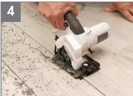
4 Carefully cut along the perimeter marks you made.
