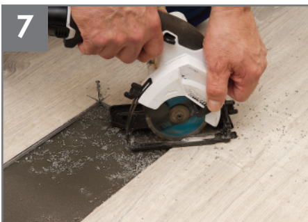
7 Carefully cut the diagonals. Vacuum up the debris.
