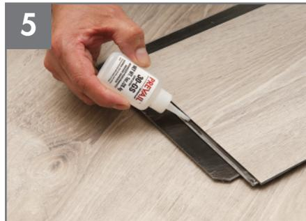
Apply a scant bead of Prevail™ 30-GS to the groove sides of the replacement plank.
