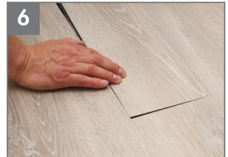
Align the cut corner first, then drop the replacement plank into position.
