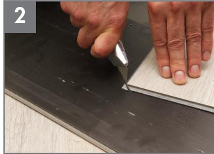
Cut off the corner where the two grooved edges meet.
