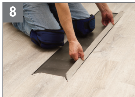
8 Remove the remaining strips of material from the long and short edges.
