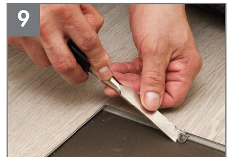
9 Remove the lock from the long and short edges of the surrounding material with a small chisel. Vacuum up debris.
