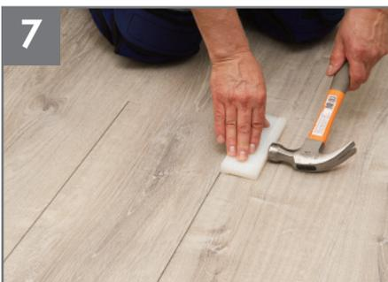
Use the Prevail™ Tapping Block on the long and short sides to ease the replacement plank into place. Hand roll the joints.
